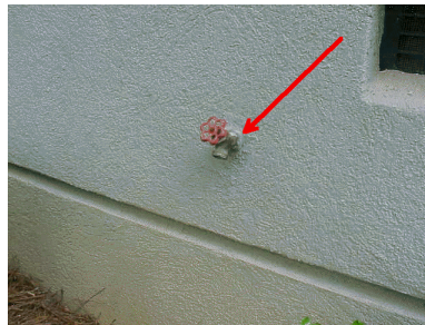
Seal all utility breaches
