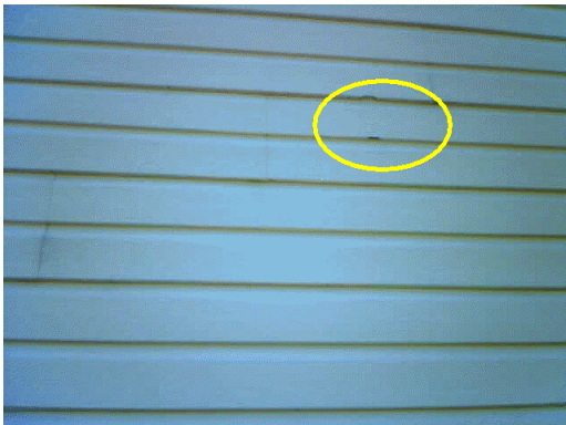
Replace all damaged siding along the rear of the home and on the chimney chase.
